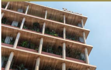
GOOD CYCLE BUILDING 001 by Nori Architects and Asanuma Corporation
